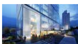
Nidakule Atasehir / Istanbul, TURKEY Standby 7x774 kVA Synchronized Diesel Generator Sets
