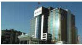
Eregli Hospital / Konya, TURKEY Standby 4x1130 kVA Diesel Generator Sets
