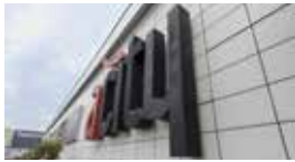
Acity Outlet Center Project / TURKEY 4x500 kWe Trigeneration System
