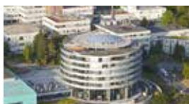
EMBL Heidelberg Biology Institute / GERMANY Standby 1x1000 kVA Diesel Generator Set
