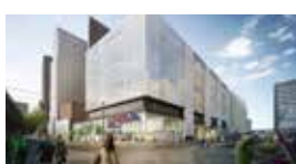
ING Haagse Poort / HOLLAND Standby 2x385 kVA Synchronized Diesel Generator Sets
