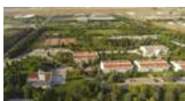
Tusas Engine Plant / Eskisehir, TURKEY Standby 1x1650 kVA Diesel Generator Set
