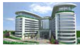
Buyukcekmece Hospital / Istanbul, TURKEY Standby 2x2025 kVA Diesel Generator Sets
