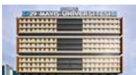
Istanbul 29 Mayıs University / Istanbul, TURKEY Standby 2x721 kVA Synchronized Diesel Generator Sets
