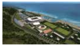
Trabzon Akyazi Stadium / Trabzon, TURKEY Standby 1x1900 kVA, 1x2065 kVA, 1x2200 kVA Diesel Generator Sets
