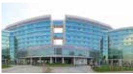
Malatya Hospital / Malatya, TURKEY Standby 4x1900 kVA Diesel Generator Sets
