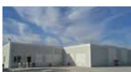
Calik Enerji aSt 2 - Diesel Generator / TURKMENISTAN Standby 3x116 kVA, 4x500 kVA Synchronized Diesel Generator Sets
