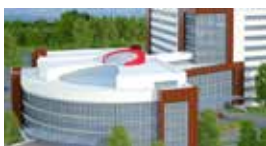
Kepez 300 - Bed State Hospital / Antalya, TURKEY Standby 4x1650 kVA Synchronized Diesel Generator Sets 2x400 kW Trigeneration system
