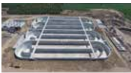
Manisa Waste Water Treatment Plant / Manisa, TURKEY Standby 1x2500 kVA Diesel Generator Set
