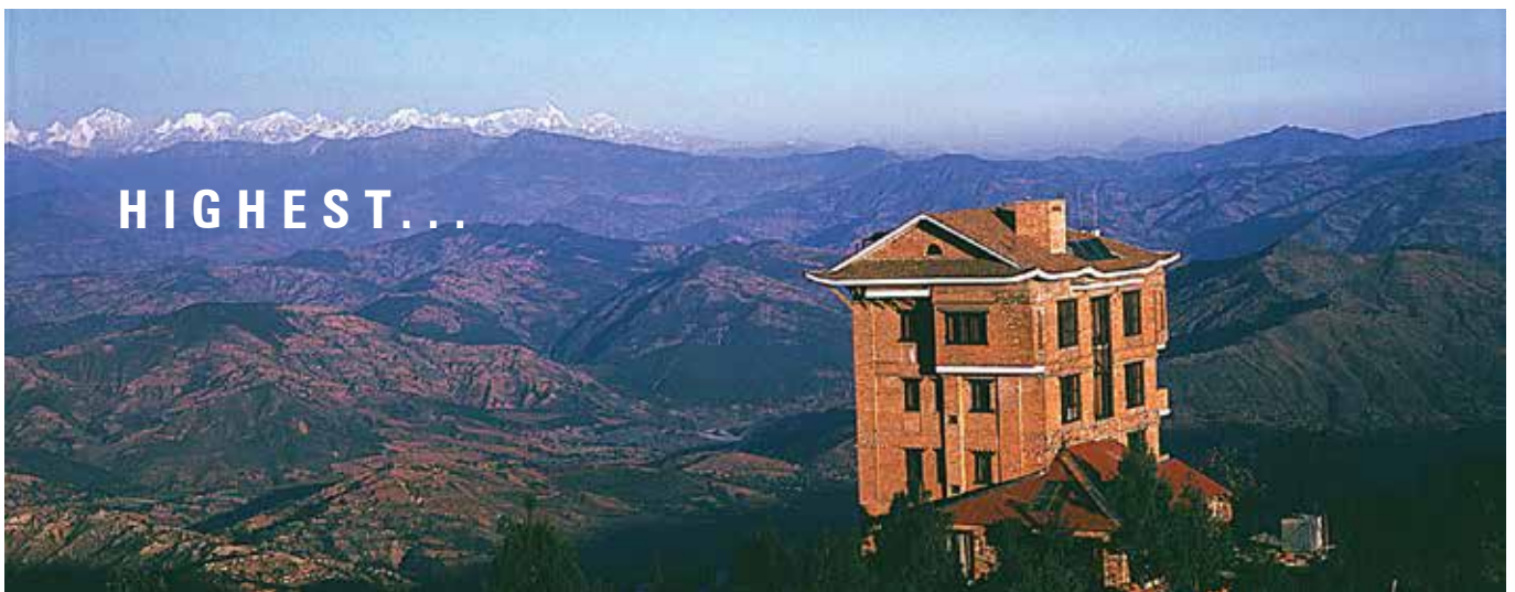
Fort Resort Hotel / Nepal (Altitude of 2.200 meters) 1x180 kVA Diesel Generator Set
