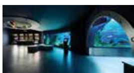
Istanbul Aquarium / Istanbul, TURKEY Standby 1x1500 kVA, 1x1900 kVA Diesel Generator Sets
