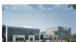
Doğuş Oto Kartal Plaza / Istanbul, TURKEY Standby 4x552 kVA Synchronized Diesel Generator Sets
