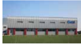
Embil Cerkezkoym Pharmaceutical Factory / Tekirdag, TURKEY Standby 3x905 kVA Synchronized Diesel Generator Sets
