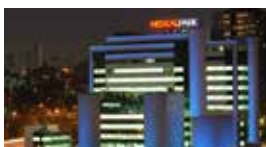
Medical Park Goztepe / Istanbul, TURKEY Standby 3x715 kVA, 2x775 kVA Synchronized Diesel Generator Sets
