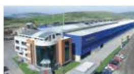
Kardemir A.S. / Karabuk, TURKEY Standby 2x1110 kVA Synchronized Diesel Generator Sets
