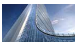
Istanbul Sapphire / TURKEY Standby 2x2100 kVA AUTO Synchronized Diesel Generator Set Standby 2x1425 kVA Synchronized Diesel Generator Set
