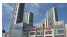
Brandium Hotel-Residence-Shopping Mall / Istanbul, TURKEY Standby 22x774 kVA, 4x660 kVA Synchronized Diesel Generator Sets
