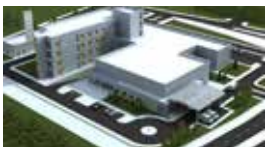
Sinop Hospital / Sinop, TURKEY Standby 2x880 kVA Diesel Generator Sets
