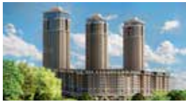
Trendist Atasehir Community Buildings / Istanbul, TURKEY Standby 3x1130 kVA, 2x905 kVA, 3x631 kVA Synchronized Diesel Generator Sets
