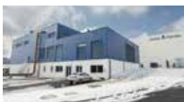
Santa Farma Pharmaceutical Factory / Istanbul, TURKEY Standby 3x2500 kVA Synchronized Diesel Generator Set
