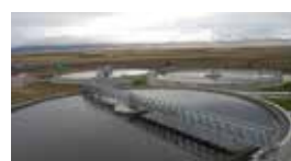
Erzurum Treatment Plant / Erzurum, TURKEY Standby 1x1400 kVA, 1x200 kVA Diesel Generator Set
