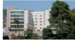
Sariyer Hospital / Istanbul, TURKEY Standby 4x1130 kVA Diesel Generator Sets
