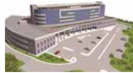
Beylikduzu Hospital / Istanbul, TURKEY Standby 3x1130 kVA Diesel Generator Sets
