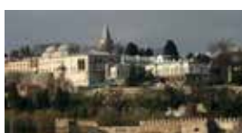
Topkapi Palace / Istanbul, TURKEY Standby 1x424 kVA Diesel Generator Set
