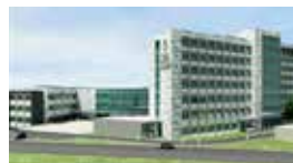
Tuzla State Hospital / TURKEY 2x400 kW e Trigeneration System
