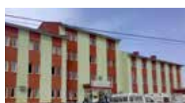
Kagizman State Hospital / Kars, TURKEY Standby 2x880 kVA Diesel Generator Sets
