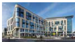
Southmead Hospital / ENGLAND Standby 2x1035 kVA Diesel Generator Set
