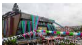
Darica Park AVM / Izmit, TURKEY Standby 3x657 kVA Synchronized Diesel Generator Sets
