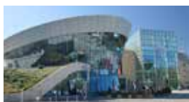
Dostyk Plaza / KAZAKHISTAN Standby 2x2025 kVA Diesel Generator Set
