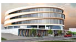
Vakifbank Sports Hall / Istanbul, TURKEY Standby 2x1400kVA Synchronized Diesel Generator Set
