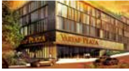
Varyap Pendik Plaza / Istanbul, TURKEY Standby 3x1100 kVA Synchronized Diesel Generator Sets
