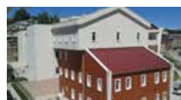
Tercan State Hospital / Erzurum, TURKEY Standby 1x1900 kVA Diesel Generator Sets
