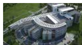
Erzurum Sultan Murat I State Hospital / TURKEY 2x430 kW Trigeneration System
