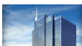
Maslak Kar Plaza / Istanbul, TURKEY Standby 2x1600 kVA Synchronized Diesel Generator Sets
