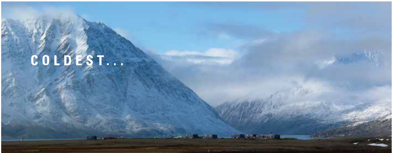
Zackenberg Research Institute / Greenland Standby 1x27 kVA 0°C cold start Auto Diesel Generator Set
