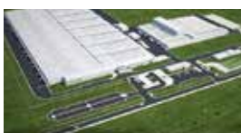
A.Özcan Rubber Factory / Ankara, TURKEY Standby 2x750 kVA Diesel Generator Sets
