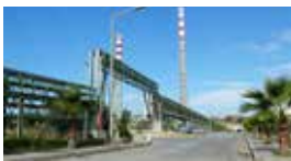
Anadolu Glass Factory / Mersin, TURKEY Standby 2x2280 kVA Automatic Diesel Generator Sets
