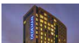
Bostanci Dedeman Hotel / Istanbul, TURKEY Standby 4x1130 kVA Synchronized Diesel Generator Sets
