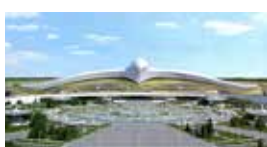
New Ashgabat International Airport / TURKMENISTAN Standby 4x1265 Kva Synchronized Diesel Generator Sets
