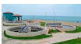
HATSU Hatay Water Treatment Plants / Hatay, TURKEY 42 units of standby Diesel Generator Sets at various powers
