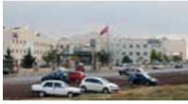
Aksaray Hospital / Aksaray, TURKEY Standby 4x1650 kVA Diesel Generator Sets
