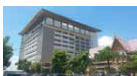
Thailand Raiking Hospital / THAILAND Standby 1x1900 kVA Diesel Generator Set
