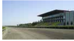
Sanliurfa Race Course / Sanliurfa, TURKEY Standby 5x778 kVA Diesel Generator Sets
