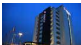
Sekerpinar Ramada Hotel / Izmit, TURKEY Standby 2x1000 kVA Synchronized Diesel Generator Sets
