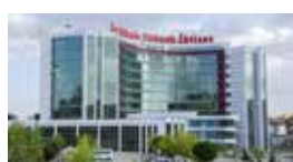
Kirkkale High Specialized Hospital / Kirkkale, TURKEY Standby 5x721 kVA Diesel Generator Sets
