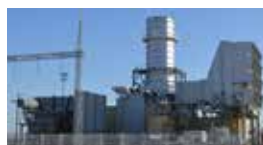
Ahal - Derweze Gas Turbine Plant / TURKMENISTAN Standby 4 x1400 kVA Black Start featured Diesel Generator Sets
