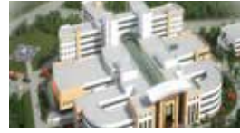
Corum State Hospital / Corum, TURKEY Standby 3x1130 kVA, 2x1425 kVA, 1x1650 kVA Diesel Generator Sets
