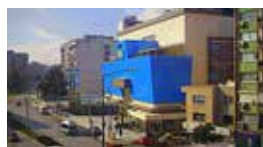
Izmir Park Shopping Mall / Izmir, TURKEY Standby 4x778 kVA Synchronized Diesel Generator Sets
