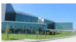
Hatay Hospital / Hatay, TURKEY Standby 5x1900 kVA Diesel Generator Sets
