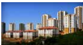
Kayabasi Housing Project / Istanbul, TURKEY Standby 4x880 kVA, 4x552 kVA Diesel Generator Sets
