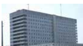
Pinsk Hospital / BELARUS Standby 2x275 kVA Diesel Generator Set
