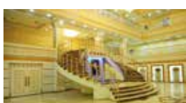
Presidency of Turkmenistan / TURKMENISTAN Standby 1x1000 kVA Diesel Generator Set
