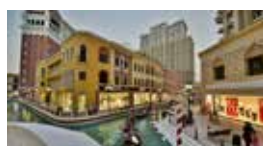
Viaport Venezia / Istanbul, TURKEY Standby 7x750 kVA, 10x560 kVA, 8x750 kVA Synchronized Diesel Generator Sets
