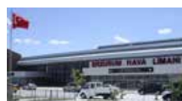
Erzurum Airport / Erzurum, TURKEY Standby 2x1125 kVA Synchronized Diesel Generator Sets
