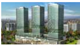
Istanbul 216 Community Buildings / Istanbul, TURKEY Standby 2x880 kVA Synchronized Diesel Generator Sets
