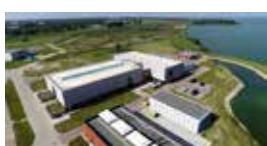
Andjik-III Drinking Water Production Plant Project / HOLLAND Standby 4x2200 kVA Synchronized Diesel Generator Sets
